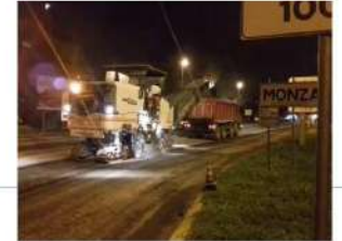
Works for asphalt laying started on 17 September 2018
