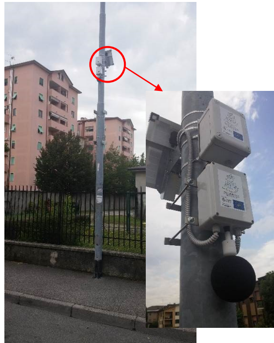
Figure 4. Example of sensor installed on a light pole.
