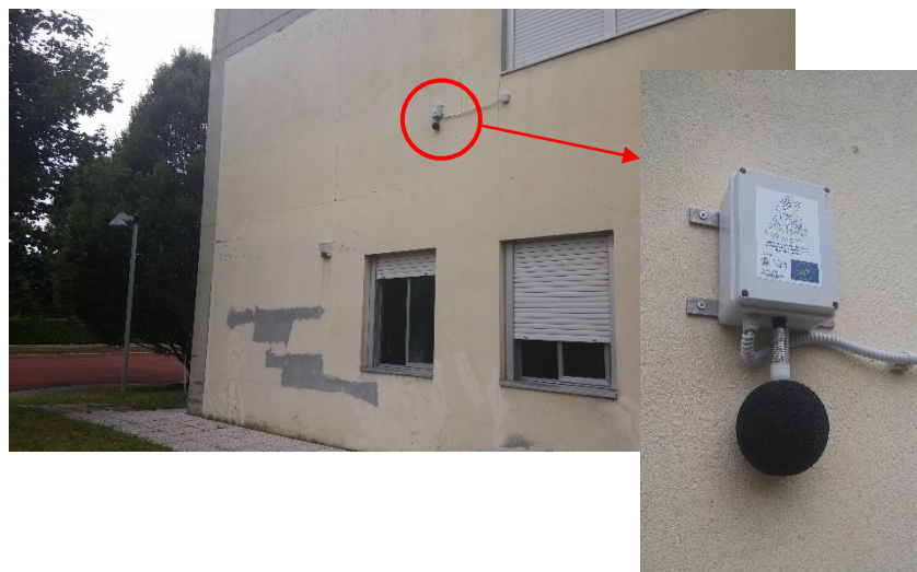
Figure 3. Example of sensor installed on the façade of a public building.
