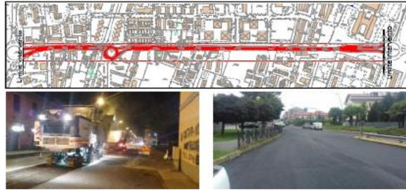
Figure 1 – Area of the intervention for the laying of dense-graded low-noise paving in Viale Libertà
