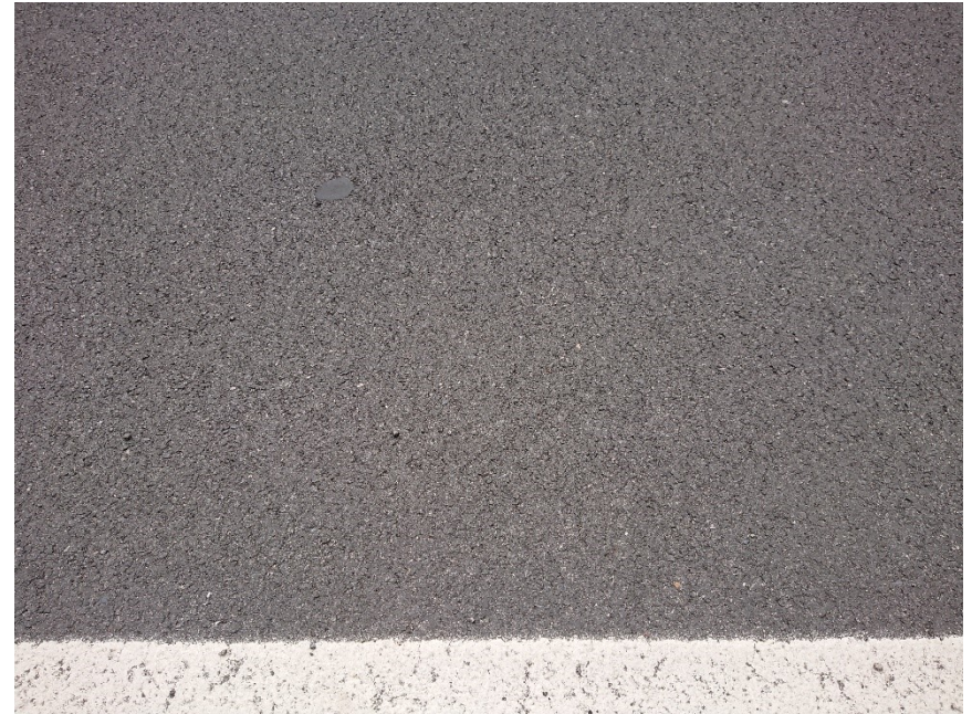
Particular weaving of the wear layer 'Dense Graded'
