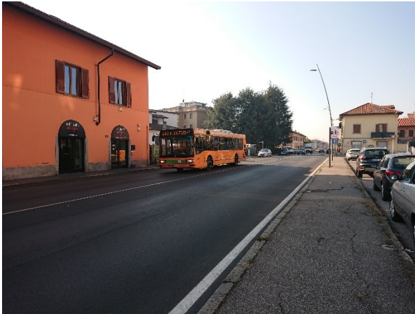
Condition of the pavement 4 months after the laying
