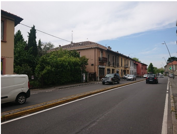
Condition of the pavement 8 months after the laying
