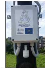
Figure 2: Smart-noise monitoring system
