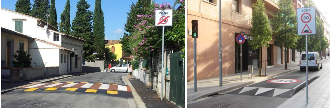
Figure 15 – Example of 30 km/h zone
