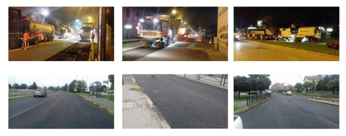
Figure 1 – Spreading of low noise asphalt.
